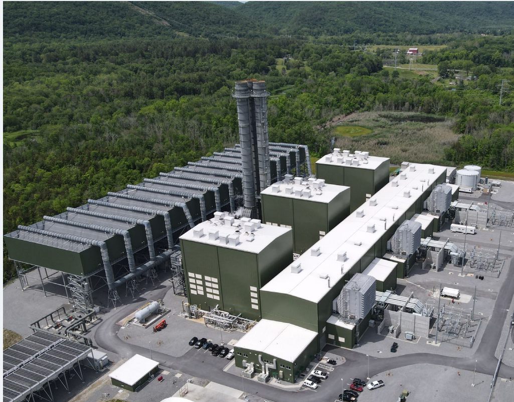
Cricket Valley will undertake a demonstration project, starting in late 2022, by running a 7F.05 turbines on a blend of natural gas with 5% "green hydrogen" by volume
